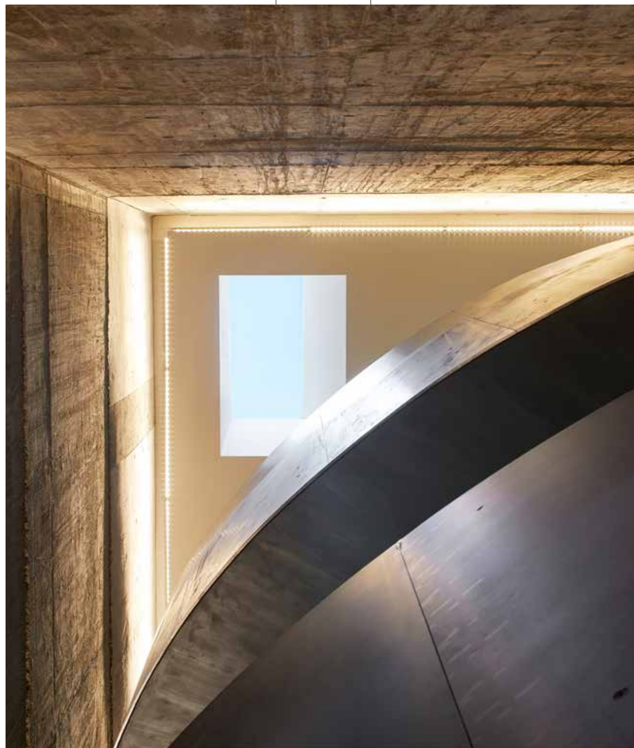
Stella McCartney's 23 Old Bond Street store features a sculptural steel staircase and skylight. Photography by Hufton + Crow.
